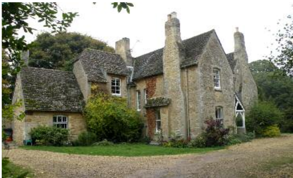
Steeple Barton Vicarage
